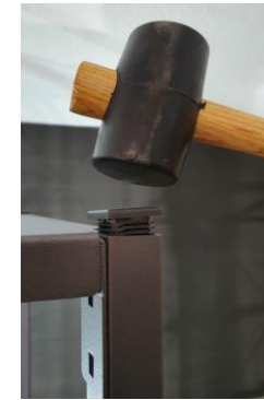
7. 4 Einsteckbuchsen einschlagen Montage der Flaschenauflage laut Folgeseite Xi Rack Anbau direkt an Basis anbauen 7. Mounting of 4 plastic caps Mounting of bottle rests as described on following page, Xi Rack Extension can be added directly on Basic Rack
